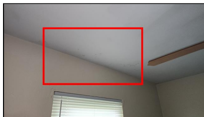
3.0 Item 4(Picture) Example/ Sample- 6- Rear Bedroom
