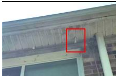
7.2 Item 1(Picture) Example/ Sample- rear of building
