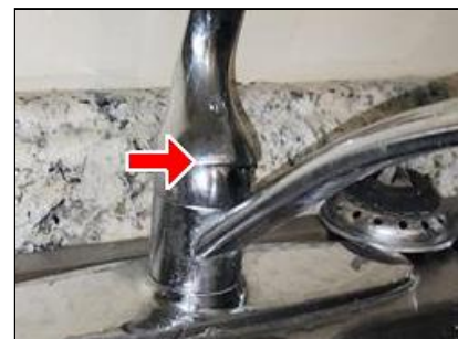
5.4 Item 6(Picture) Example/ Sample- 6- Kitchen Sink- water control handle leaks while in use if pressure applied to handle
