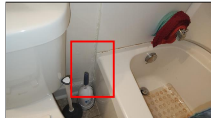
3.0 Item 3(Picture) Example/ Sample- 8- Bathroom
