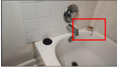
3.0 Item 15(Picture) Example/ Sample- 1- Bathroom Shower
