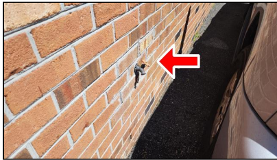
5.4 Item 10(Picture) Example/ Sample- Right side of building
