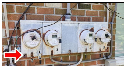
6.3 Item 5(Picture) Example/ Sample- meter box "1"- opening
