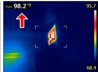
7.0 Item 3(Picture) Example/ Sample- Unit 5- heat supply at time of inspection unit number
