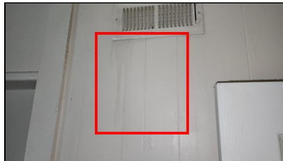
3.0 Item 1(Picture) Example/ Sample- 7- Rear Left Bedroom
