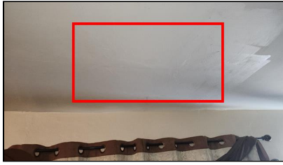
3.0 Item 7(Picture) Example/ Sample- 1- Living Room
