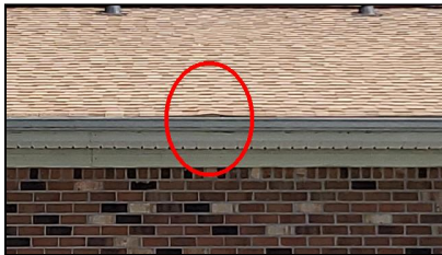
1.0 Item 1(Picture) Example/ Sample- front of building – slightly lifted risen shingle
