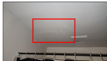
3.0 Item 6(Picture) Example/ Sample- 3- Bathroom
